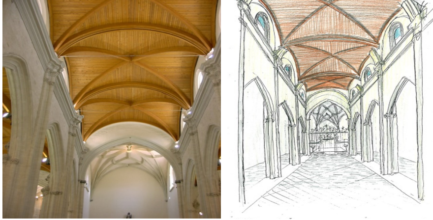
Fig. 8 Nave vaults. Photo and sketch of the design phase by the author
