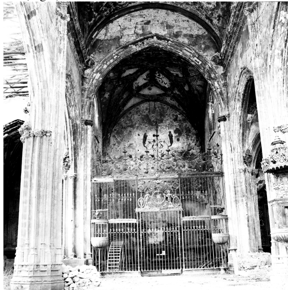
Fig. 6 State after the fire and destruction in the Civil War from 1936 to 1939. Carmelo Ruiz photo
