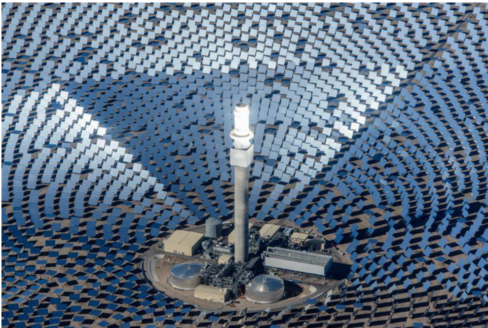
Figura 2.9. Planta Termosolar de Receptor Central (Crescent Dunes). [16]
