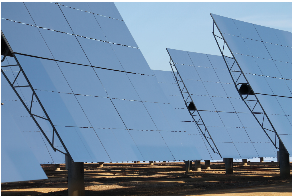
Figure 1.4: Standard heliostat design [Abengoa, 2019]
