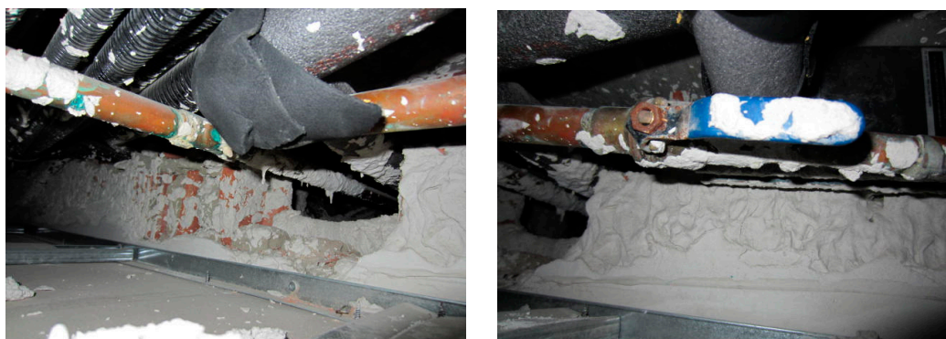
(a) Water pipe penetrations to flats from communal area service shafts
