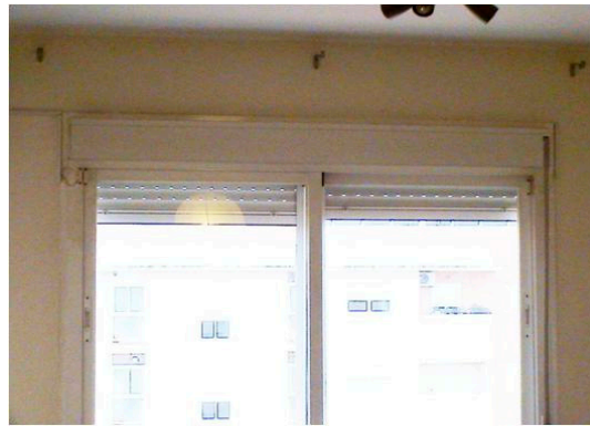
Figure 7. The window (visible spectrum) prior to the blower door test.
