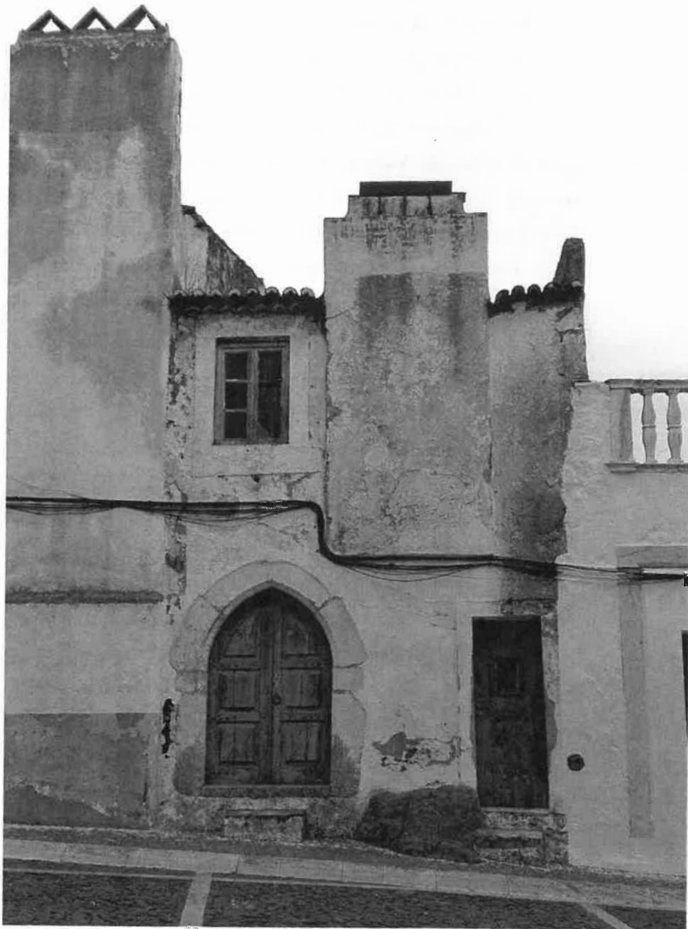
Fig. 6: Estremoz' vernacular housing inside the Castle. (Source: N/A).
