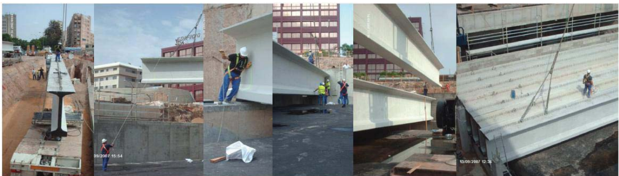
Fig. (5). Constructive process.
