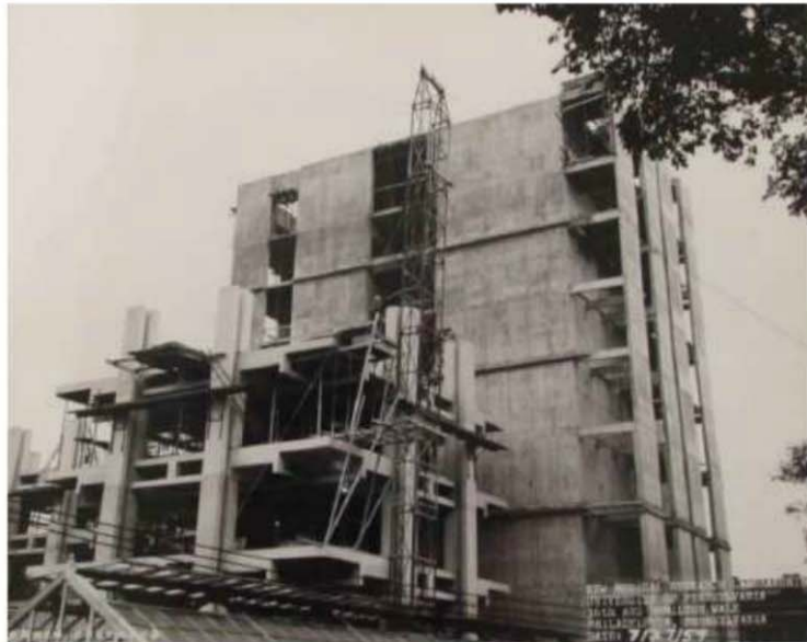
Fig. 10 Photograph that show both construction systems, the pre-fabricated pieces and the poured in site at the "X" tower. Archive No. : 030. IV.A.490.12.51.The A.A., U. of Penn.
