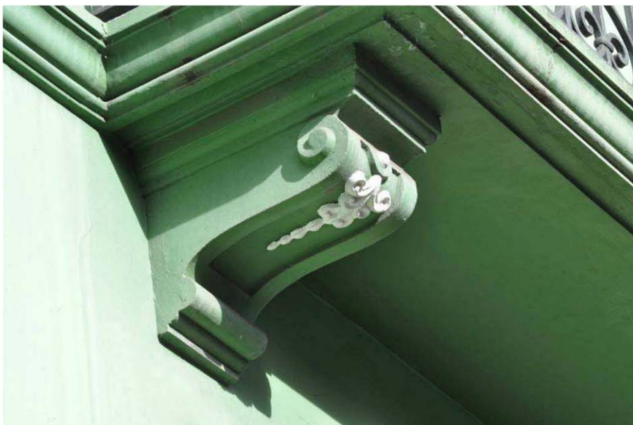
Fig. 8 Balcony bracket of the building nº 73 of Calvario Street. La Orotava
