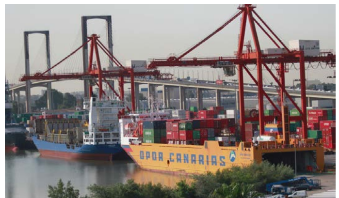
Figure 1. A view of the “Batan” dock at the Port of Seville with the container terminal at the rear.
