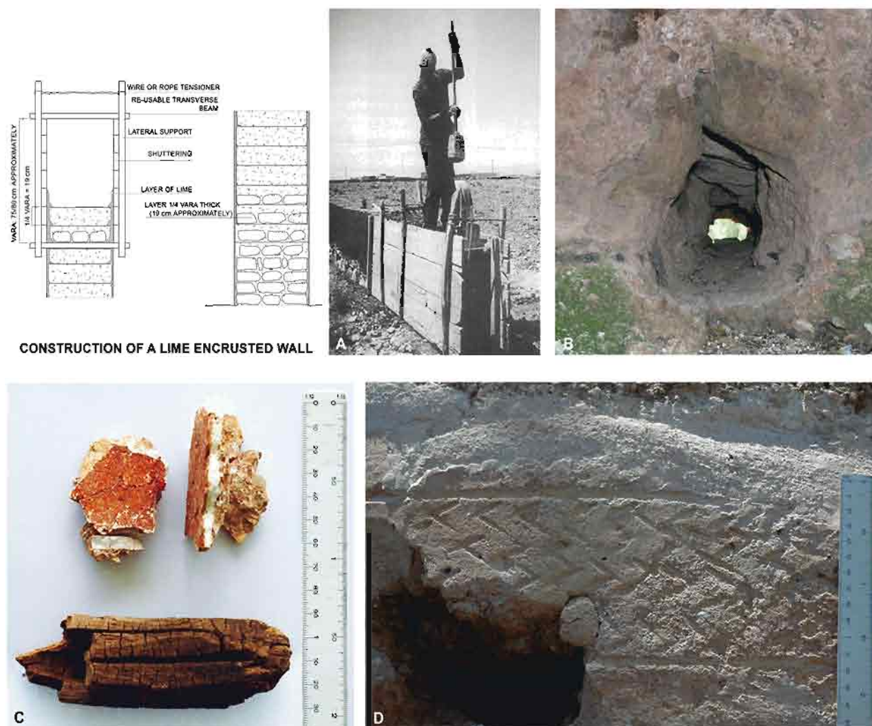
Figure 6. Shuttering design for the walls of the towers of Segura. A/ A rammed-earth wall made in Morocco. B/ A shuttered putlog hole in the towers of the Segura valley with a stone support which allowed the reuse of the horizontal timber of the rammed-earth lifts. C/ A sample of the remains of a horizontal timber and the exterior lime-encrusting of the rammed-earth wall, clearly showing its thickness. D/ Marks and geometrical designs over bands of lime applied on the rammed-earth lifts and the rows of putlog holes of the horizontal timber in the tower of Góntar .
