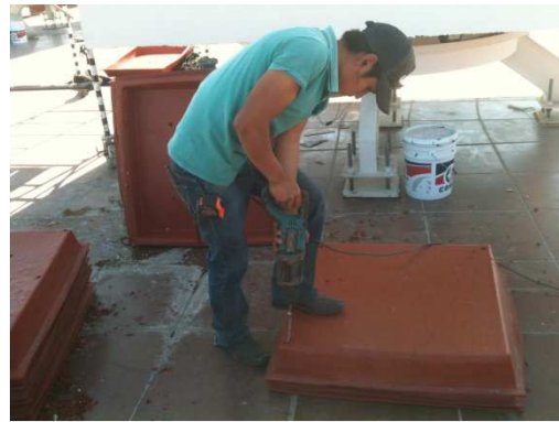
Fig. 10 "grid of holes"
