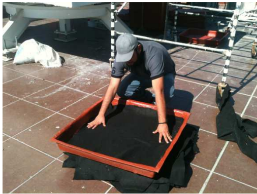
Fig. 9 "Placing geotextile"
