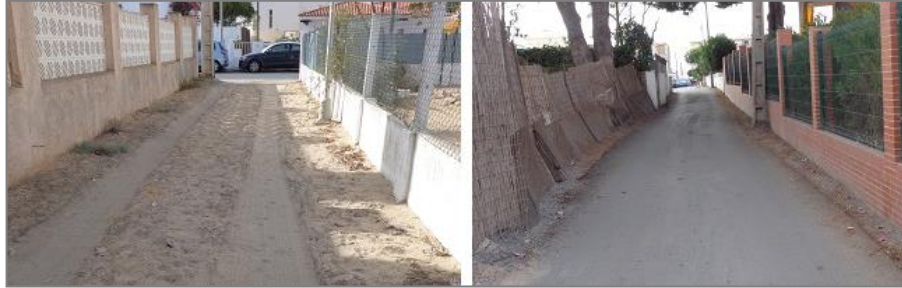
Fig. 7 Sand street with pedestrian strip and asphalt street at La Canaleta
