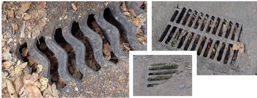
Fig. 6 Inlet grates at La Canaleta
