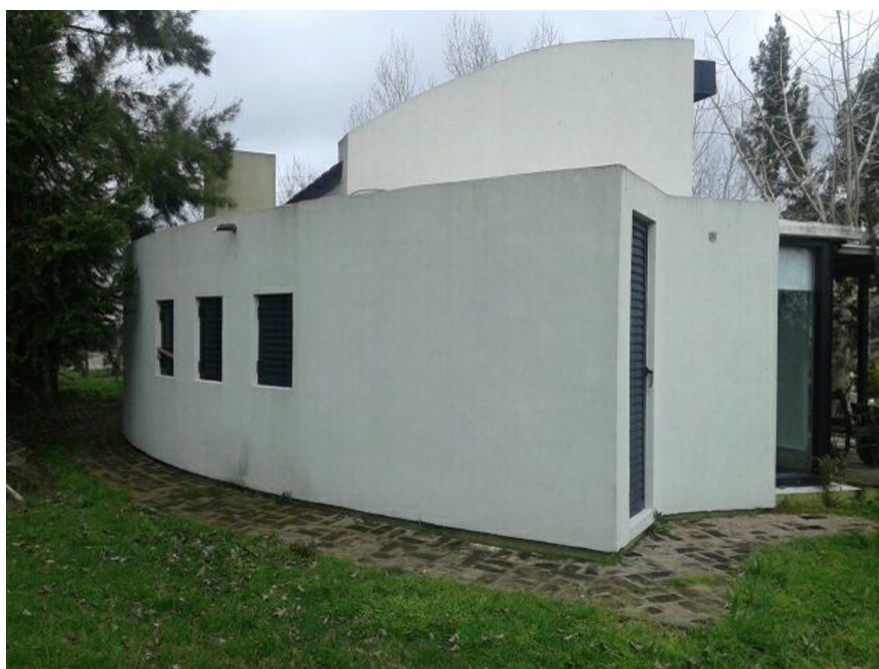
Fig. 1 Refurbished wall Southern view
