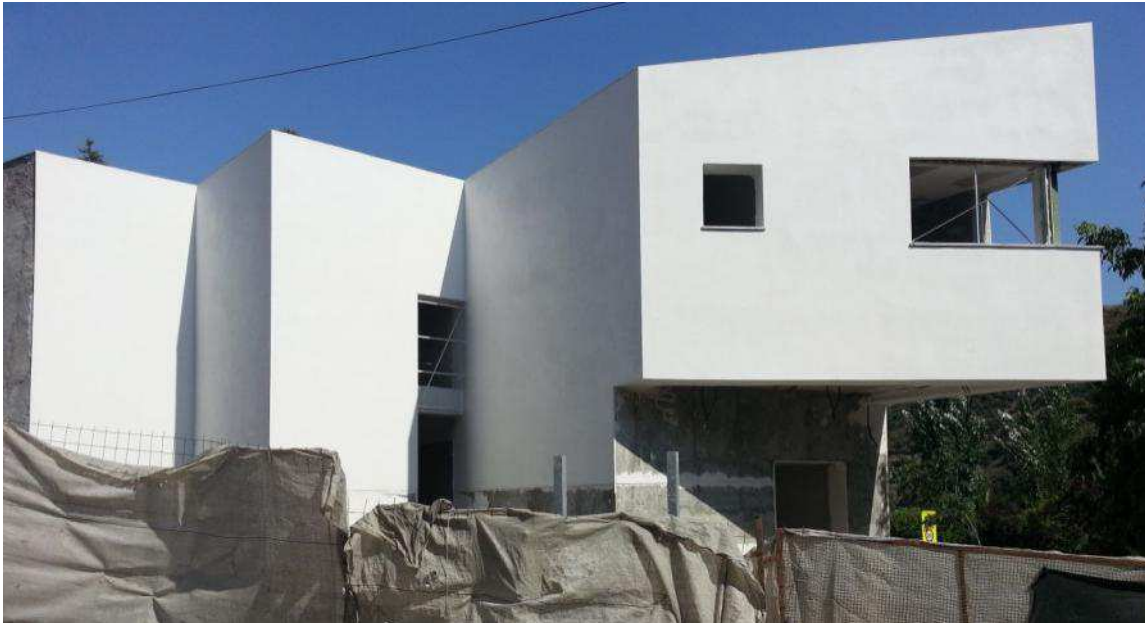
Fig. 8 “Appearance of the façades during construction. July 2013.” Source: the author.
