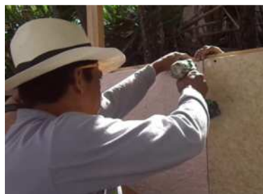
Fig. 8 “Drilling and anchorage of screws in the table boards”
