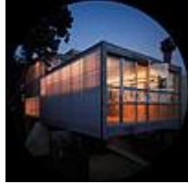
WORKHOUSE - Guthrie + Buresh Architects -1996
