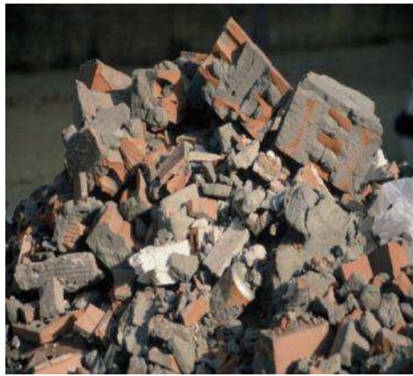
Fig. 4 “RCD generated in refurbishment”. Souce: the author.
