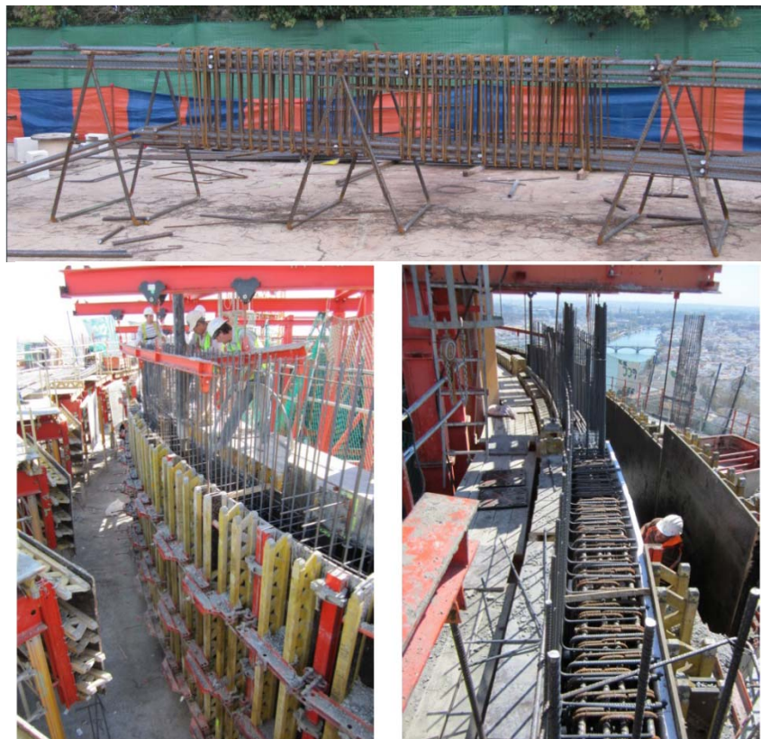
Figure 22: Reinforcement of the lintels on door gaps in the core.
