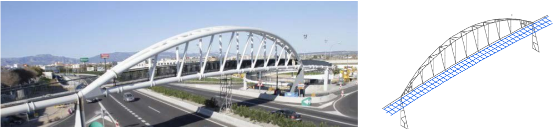
Figure 1. Footbridge under study: photograph and numerical FE model.
