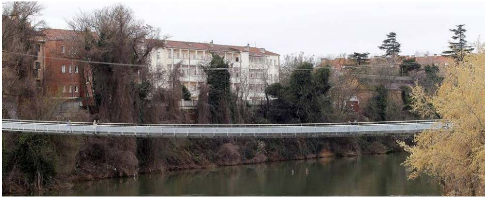
Figure 1. Pedro Gómez Bosque footbridge. Landscape view.
