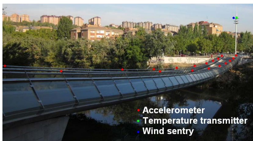
Figure 2. Monitoring system. Distribution of sensors.
