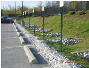
Fig.9. Cuneta Verde. (Stormwater Maintenance and Consulting, LLC)
