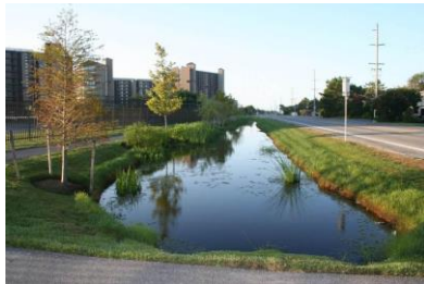
Fig.8. Cuneta verde húmeda en South Pennsylvania (U.S.A.) (Anchorage Canal Retrofit Project, 2015)
