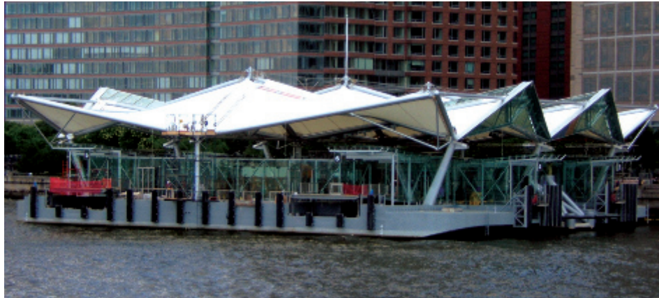
22. Battery Park City Ferry Terminal en el World Financial Center.
