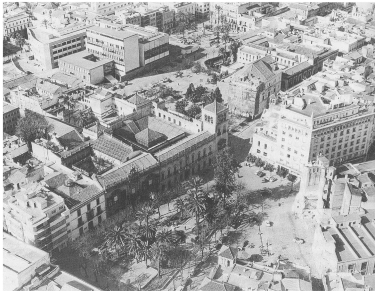
Fig. 3 The police headquarters under construction in its urban context (upper left corner) (Source: Ramón Montserrat)
