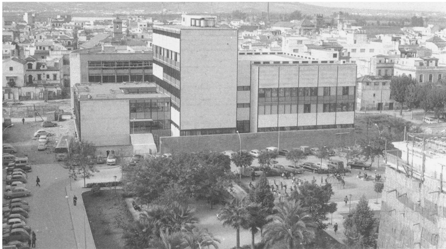
Fig. 1 Seville's former police headquarters under construction in 1964 (Source: Ramón Montserrat)
