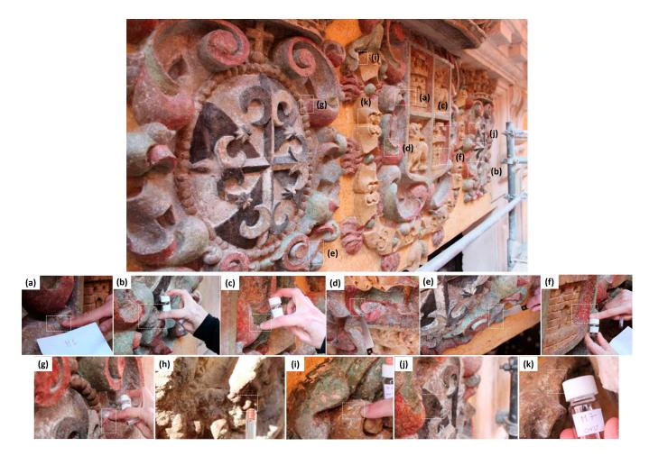
**Figure 2.** Photos of sampling zones within the façade of the Madre de Dios Convent (in white square): (a) sample 1, blue colour; (b) sample 4, green colour; (c) sample 5, green colour; (d) sample 10, green colour; (e) sample 9, turquoise colour; (f) sample 2, red colour; (g) sample 3, red colour; (h) sample 11, red-brown colour; (i) sample 6, yellow colour; (j) sample 8, black colour; and (k) sample 7, golden colour.
