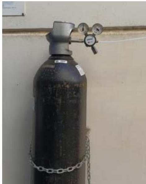
Figure 3. 8 - Nitrogen tank with the pressure reducer and the two pressure gauges
