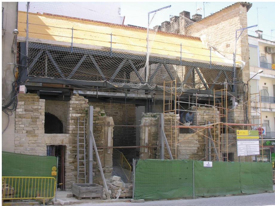
Figure 6. View of the construction process. The pieces are located exactly at the original site after careful documentation process.
