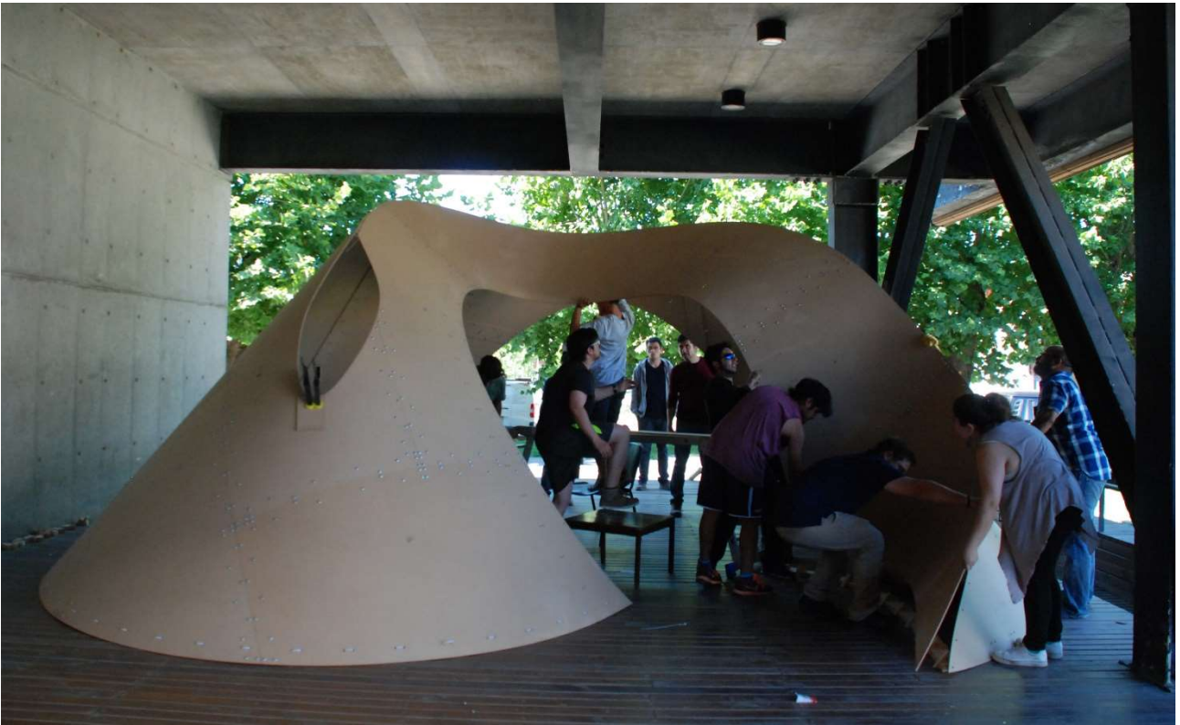
Fig. 9. Curvature and fastening of the skin along the crest of the dune and along the base beam (Source: Authors' own)
