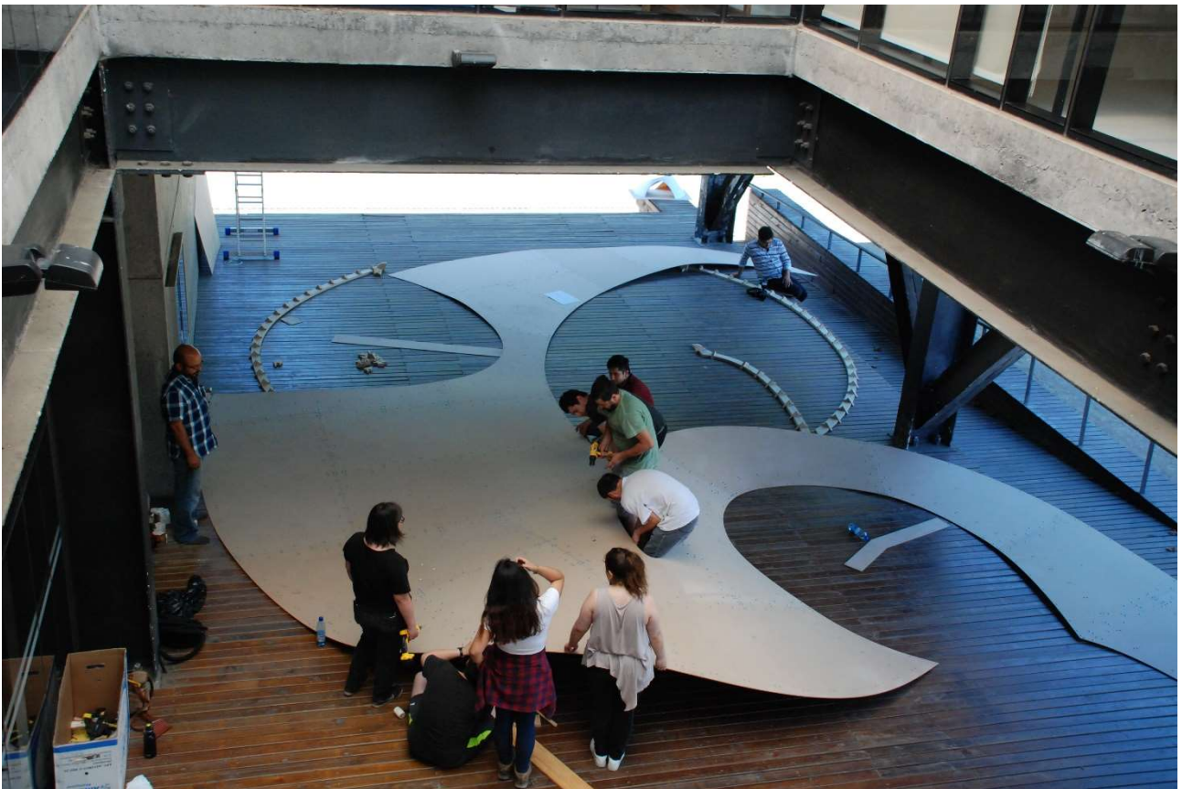
Fig. 8. Assembly of the Bio-Dune Pavilion as a single skin (Source: Authors' own)
