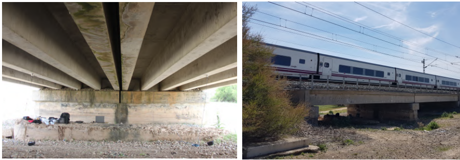
Figure 1: Old Guadiana Bridge: general view.
