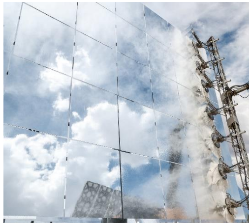
Figure 4-1 Crescent Dunes (Tonopah) Heliostat. 6x6 ft each facet, 35 facets each heliostat, total surface area of 116 m 2
