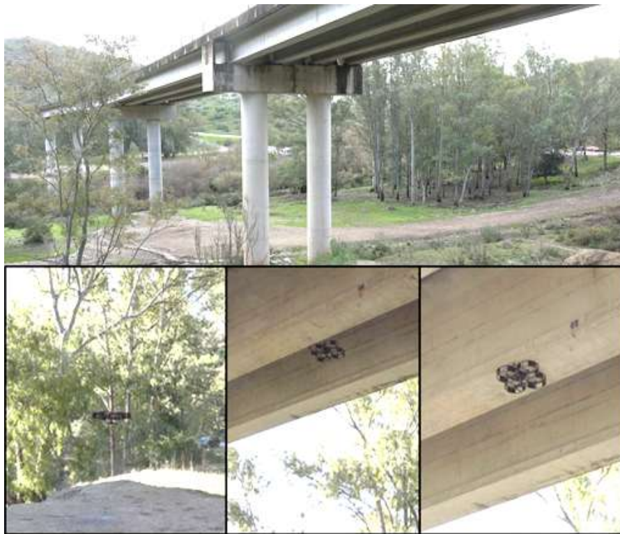
Figure 4.12: Navas bridge and experiment overview
