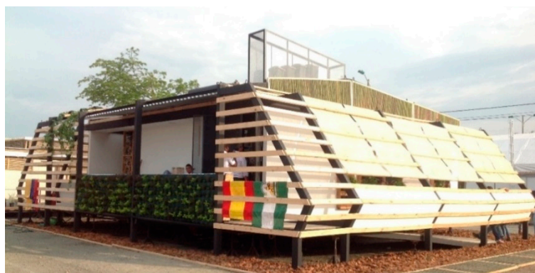
Figure 16. Photo of the north-east facade.
