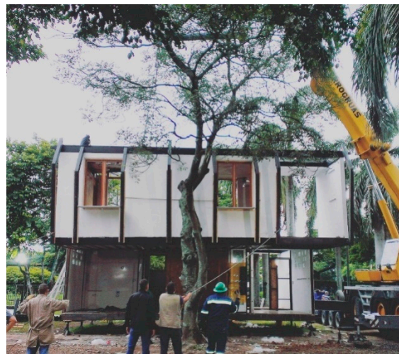
Figure 1. Image of the prototype assembly process.
