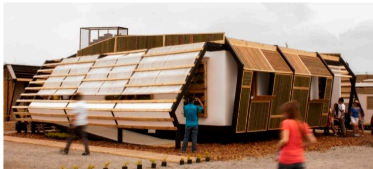
Figure 15. Photo of the south-east facade.
