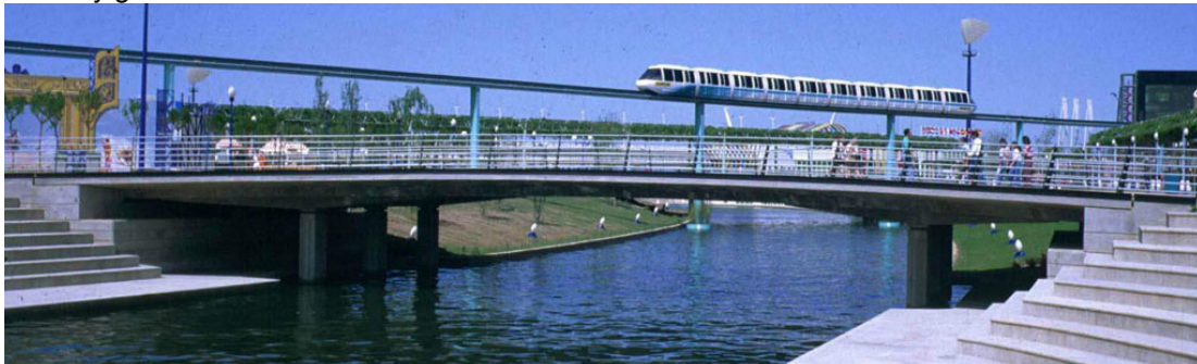
Figure 1. View of the structure.
