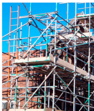
Figure 5. “Tube-and-fittings” scaffolding [10].
