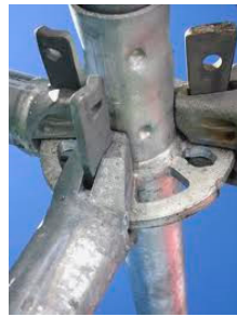
Figure 3. Joining element of multidirectional scaffolding [10].
