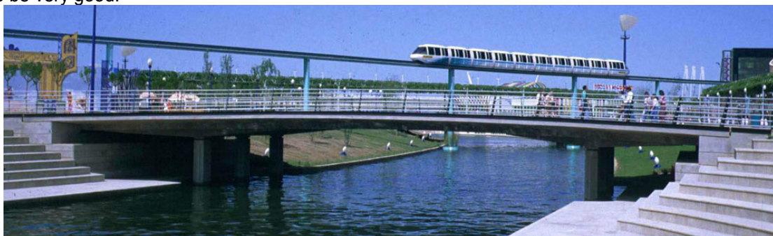
Figure 1. View of the structure.
