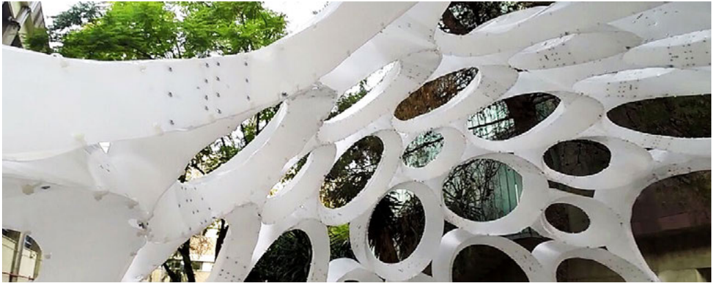
Figure 1. Photograph from the interior of the Archimedean Pavilion prototype, composed of inclined rotational parabolic domes materialised with lightweight conical components.
