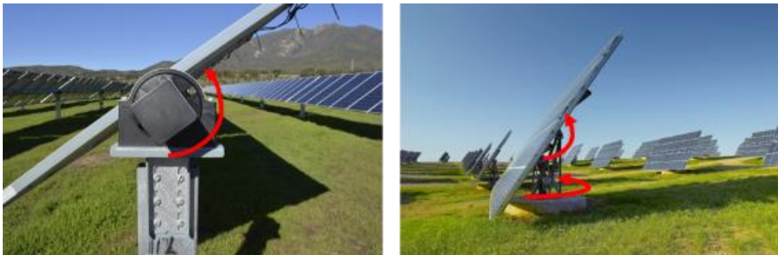
Fig. 3: 1-axis tracker (left) and 2-axis tracker (right)
