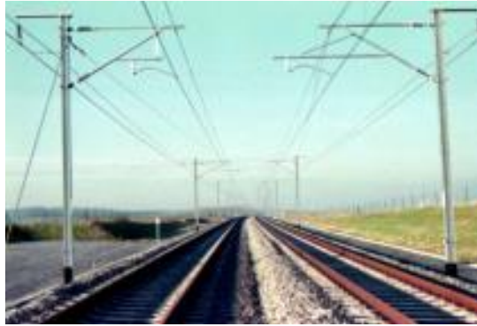
Figura 2-2 Vía del Thalys HST entre Bruselas y París. Degrande, G. 2002. “Free field vibration measurements during the passage of a Thalys high speed train”
