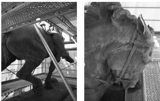
Figure 1. Formation of unstable patinas due to pollution.
