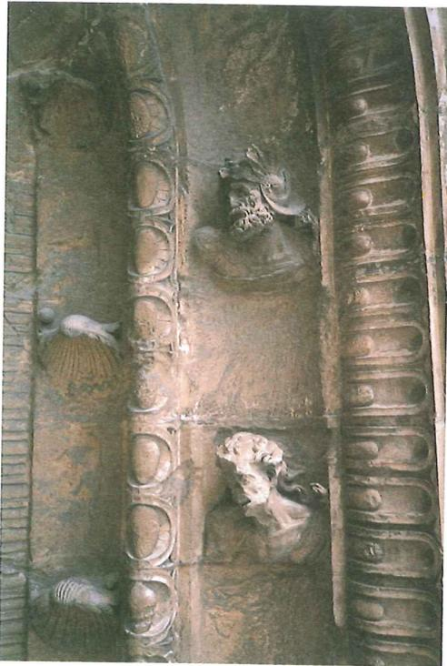
Figure 2 The effects of pollution: typical black-and-white sulphatation phenomena.
