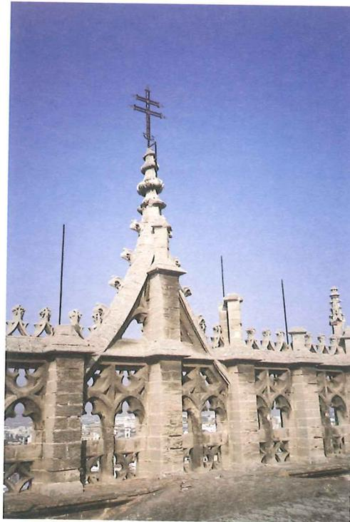
Figure 4 The effect of rusting: almost all the pinnacles higher than 2 m disappeared.
