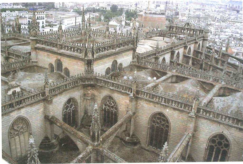
Figure 1 The extensive and flat roof of the Seville Cathedral, the main source of the problems.
