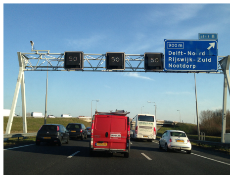
Fig. 1. VSL implementation on A13. Delft, The Netherlands.
