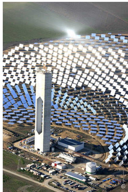
Fig. 1. Abengoa PS20: a 20Mw solar power tower
