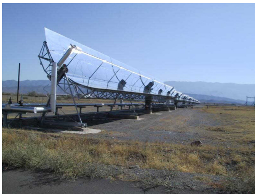
Fig. 4. DISS Parabolic trough at the Plataforma Solar de Almeria
