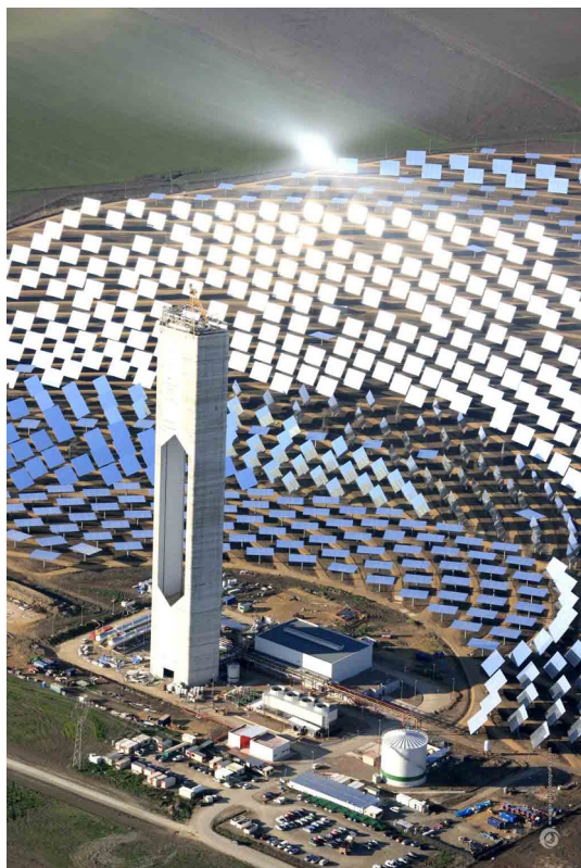
Fig. 1. Abengoa PS20: a 20Mw solar power tower
