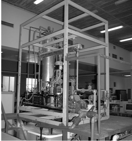
Fig. 1. Pilot plant used to apply the MMMPC.
