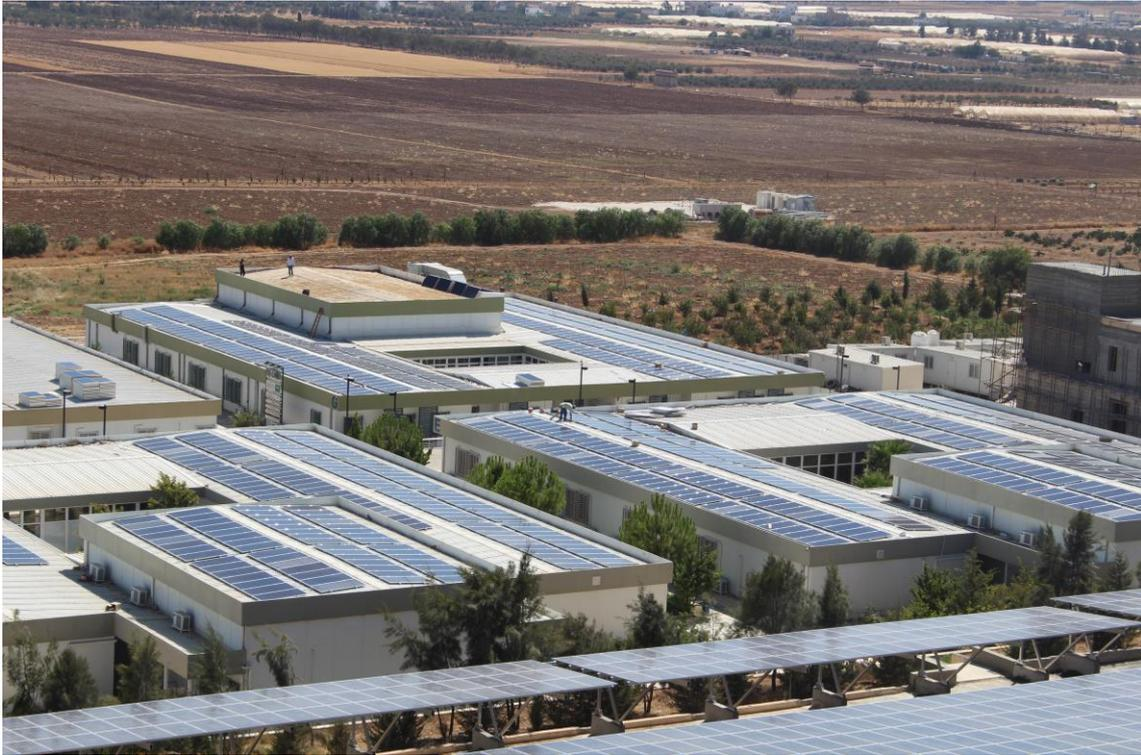
Figura 3-10. Área 6, 1256 paneles, 395.64 kW. FUENTE: [16]
