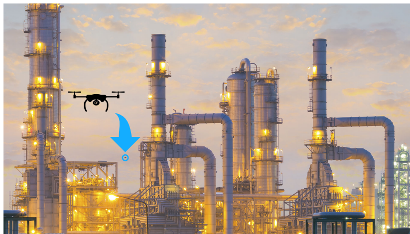
Figure 1. UAV (Unmanned Aerial Vehicle) inspection of large structures.
