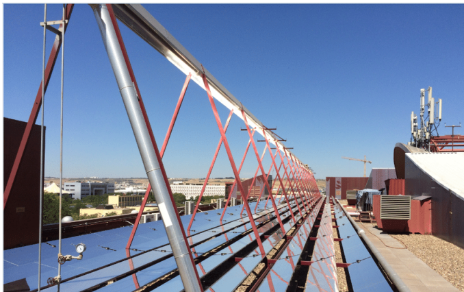
Figure 1.9: Linear Fresnel Collector solar cooling plant located at the Engineering School (ESI) of Seville
