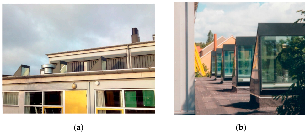
Figure 2. Final skylight proposal for Egebjerg School: (a) general view; (b) row of skylights. Source: authors. Source: authors.
