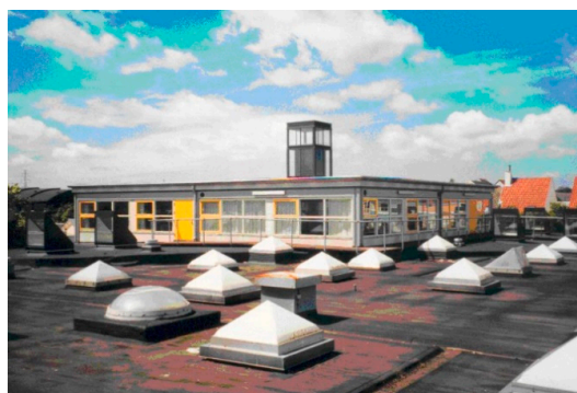
Figure 1. View of the no longer extant skylights consisting of a pyramid structure made of plastics. Source: authors.
