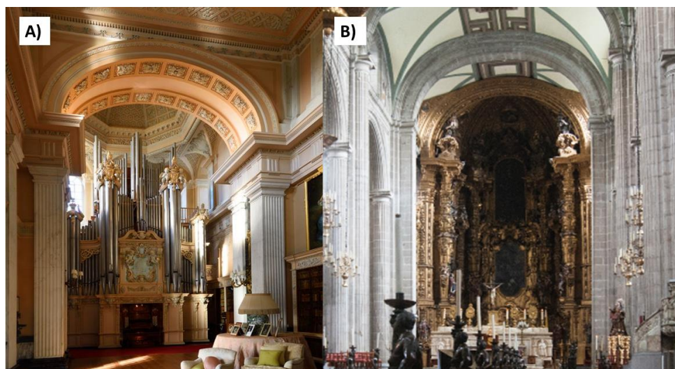
Figure 6. (A) Basket-handle arch of one of the galleries of the Blenheim Palace (UK). (B) Basket-handle arch of the central nave of the Metropolitan Cathedral of Mexico City.
