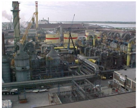
Figure 1: General view of the copper smelter [1]
