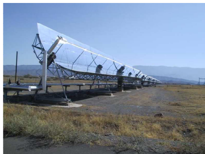
Fig. 1. DISS Parabolic Trough Solar Collector at the PSA
